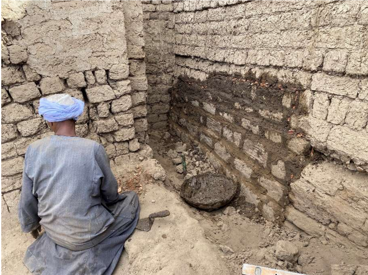
Fig. 29: Reinforcing structurally damaged walls by underpinning (photo: O. Kassab, © DAI)
