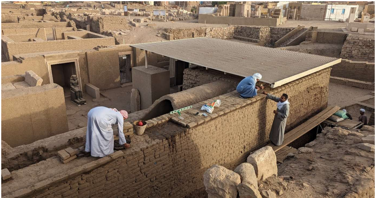
Fig. 17: Sanctuary of Heqaib, consolidation of the exterior mud-brick walls (photo: B. Ezzat, © DAI).
